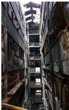
Fig. 22 The view of the stairway case with lighting clearance
