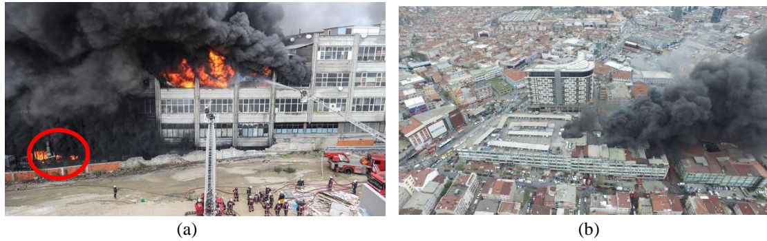
Fig. 6 The photographs of the building during the fire (NTV 2017, DNA 2017)
