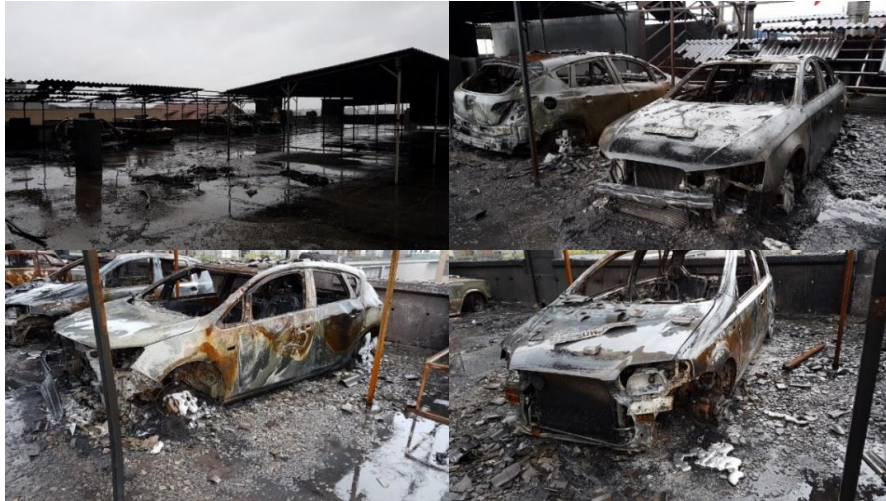
Fig. 21 Burnt vehicles that some of the aluminum wheels trims melted in the parking area on the roof
