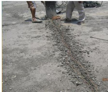
Fig. 8 Embedment of the thermocouple wire
