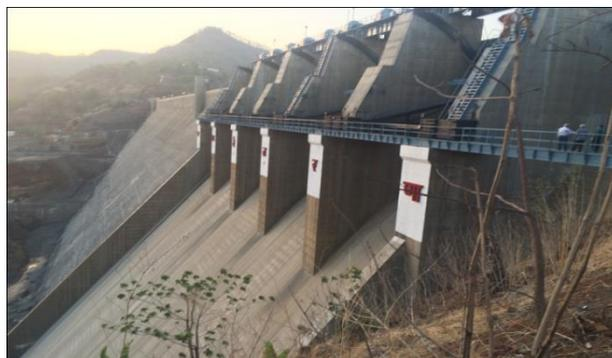
Fig. 1 Downstream view of completed 102.4m tall Middle Vaitarna RCC Dam
