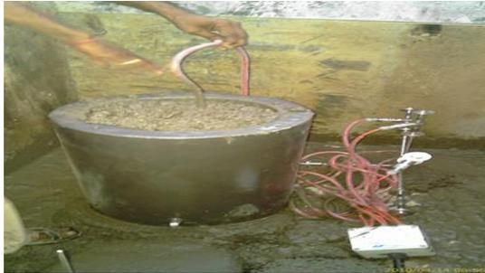
(a) Joint meter being installed
