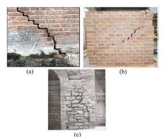
Fig. 3 The local failure mode of URM: (a) detachment failure, (b) detachment fractures alternate line of sliding, and (c) compression failure (source: Angelillo *et al.* 2014)
