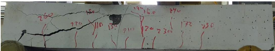
Fig. 10 Crack pattern at ultimate load for HCCS (100 mm) (Slab-3) monotonic test
