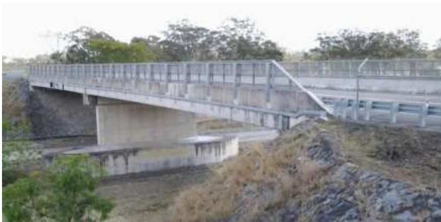
Fig. 4 A Two-span two-lane deck unit bridge
