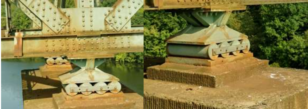
Fig. 2 Inspection of bridge roller bearings (Aibotix GmbH, 2014)
