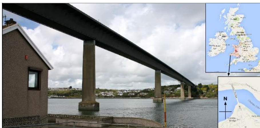
Fig. 1 The Cleddau bridge (looking from east of Pembroke dock) (left) and its geographical location (right). (Courtesy: Pembrokeshire County Council)
