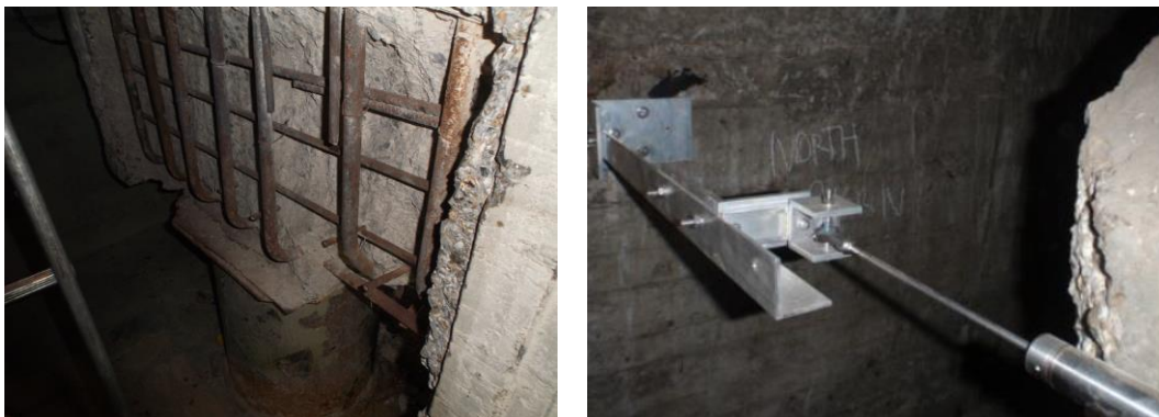
Fig. 10 Base of pier and extensometer for bearing movements
