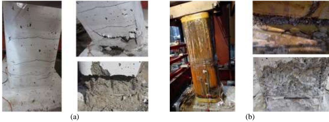
Fig. 7 Damage pattern and failure mode: (a) unconfined RC column QSS001 and (b) steel confined RC column QSS003
