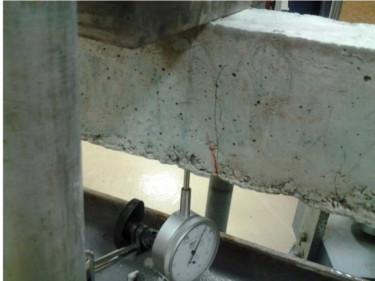
Fig. 3 Photograph of the displacement gauge and the observed damage pattern
