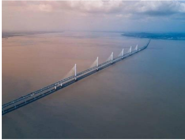
Fig. 4 Photograph of the Jiashao Bridge
