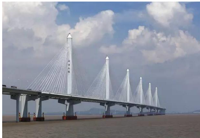
Fig. 5 Main piers of the Jiashao Bridge
