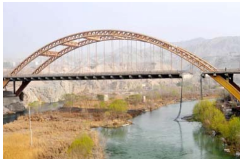
Fig. 2 The photo of collapsed Kongquehe Bridge
