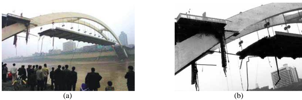
Fig.1 The photo of collapsed Nanmen Bridge
