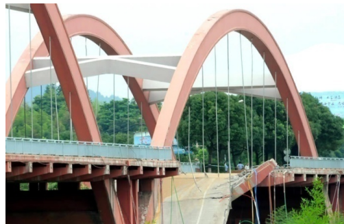
Fig. 3 One of the PLVM of the undamaged structure
