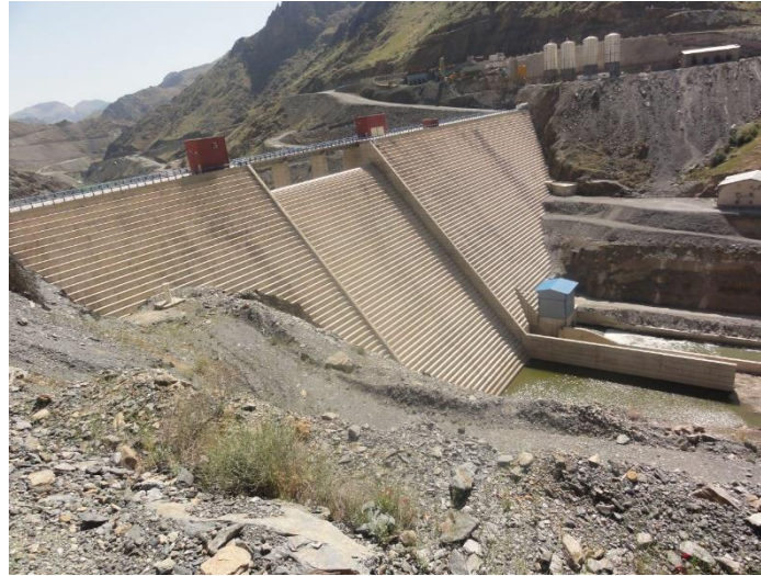
Fig. 2 View of Zhaveh dam before impounding
