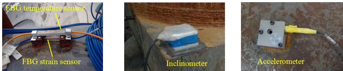
Fig. 35 Pictures of sensors installed on structure of gymnasium
