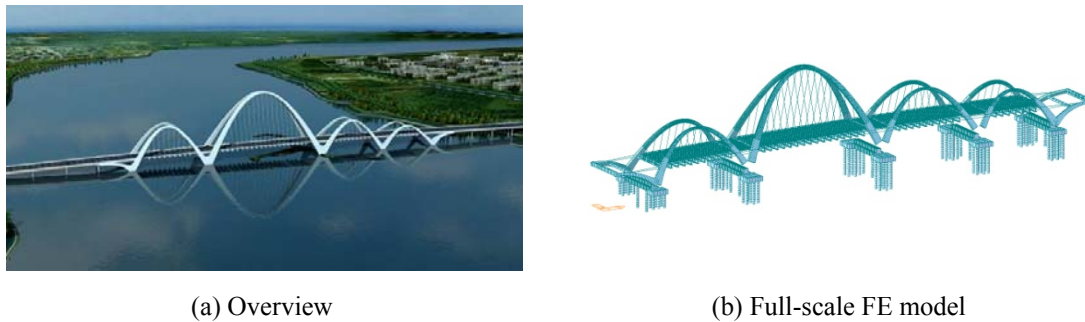
Fig. 41 Shenyang Boguan Bridge and its FE model
