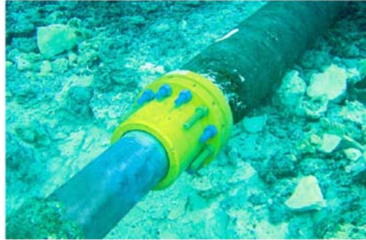
Fig. 3 Smart flange connection to 4inch pipeline on seabed
