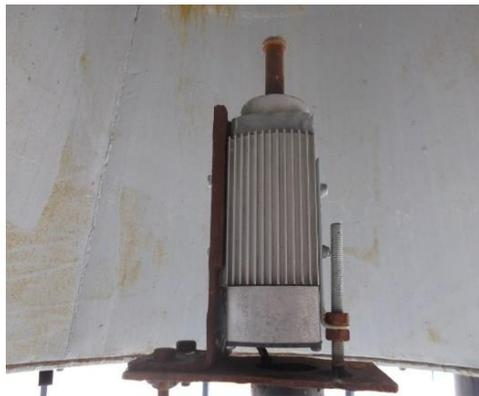
Fig. 8 The generator in the solar chimney power plants
