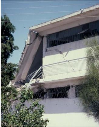
Fig. 1 Failure of short RC columns at the 1999 earthquake in Athens
