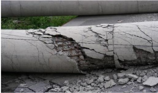
Fig. 1 Example of the bridge column failure
