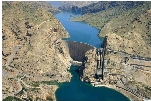
Fig. 3 Aerial view of Karoun-I double curvature arch dam
