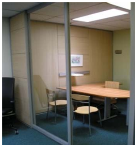
Fig. 1 Typical office space with partitions jointed to suspended acoustical ceilings
