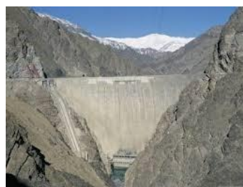
Fig. 1 Downstream view of the Karaj Dam
