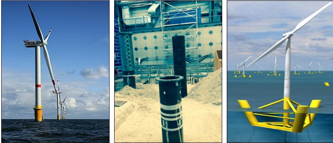
Fig. 2(a) Offshore wind turbine foundations(Wikipedia, parc éolien de Thorntonbank); (b) Foundation fatigue testing (Germany); (c) floating offshore wind turbine, Semisubmersible column (WindFloat)
