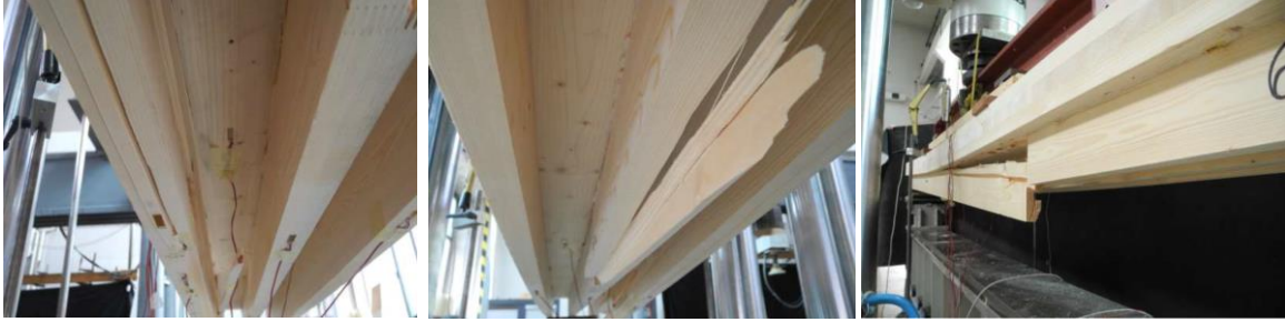
Fig. 7 Cracks in sample 6.1.a (Zisi, Aicher and Dill-Langer 2016): edge rib (left), middle rib (middle), edge rib at plate failure (right)
