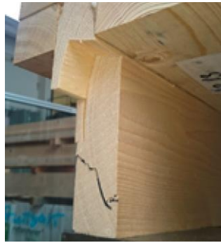
Fig. 8 Cracking systems RL-TL , modes I and II, sample 3.1.c
