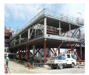
Fig. 3 Example of hanging scaffold (Hara et al. 2018a)
