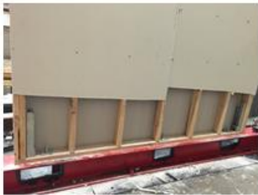
(a) Bottom of wall frame after testing
