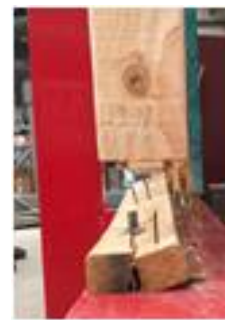
(b) Torn out OSB, fractured baseplate and combination of several failure modes
