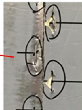
(b) Failure due to bearing of staples at the edges
