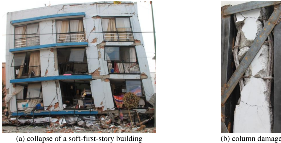
Fig. 1 Observed damage on (a) and (b)
