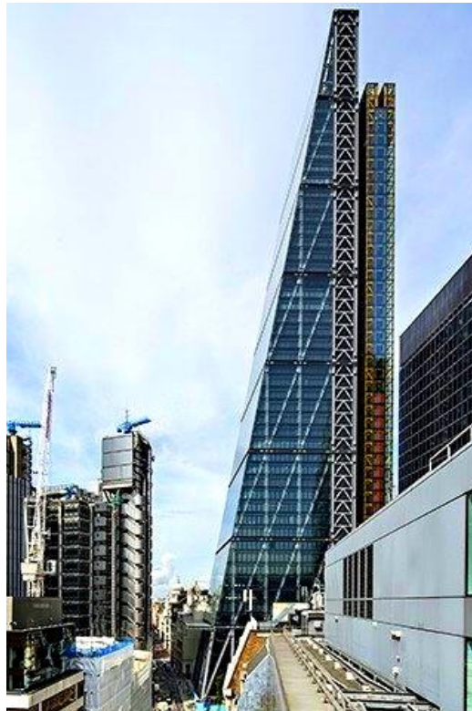
Fig. 1 Mega-scale bracing at leadenhall building in london, opened in 2014 (Levene 2014)
