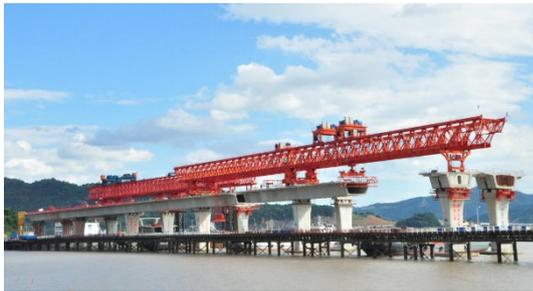
Fig. 14 Cantilever erection of the Leqing Bay Bridge
