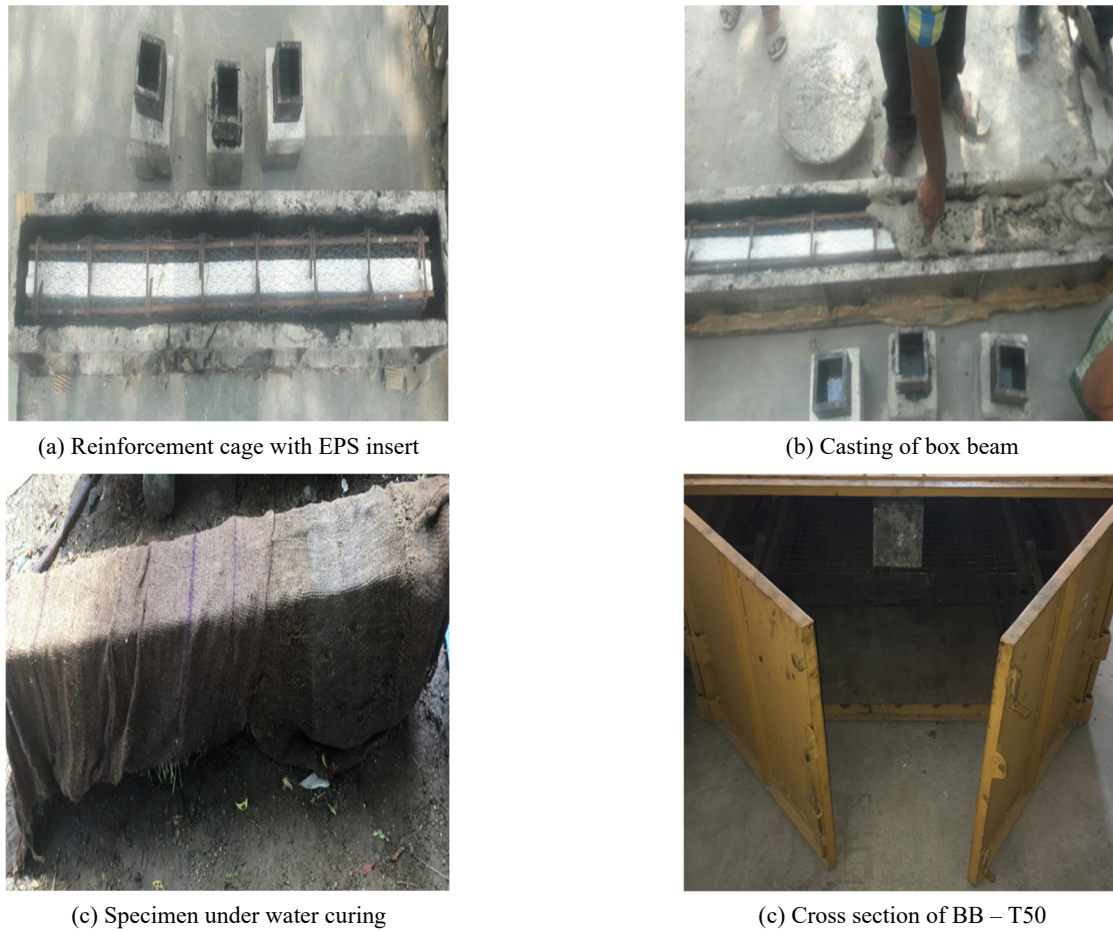
Fig. 4 Casting and curing of box beams
