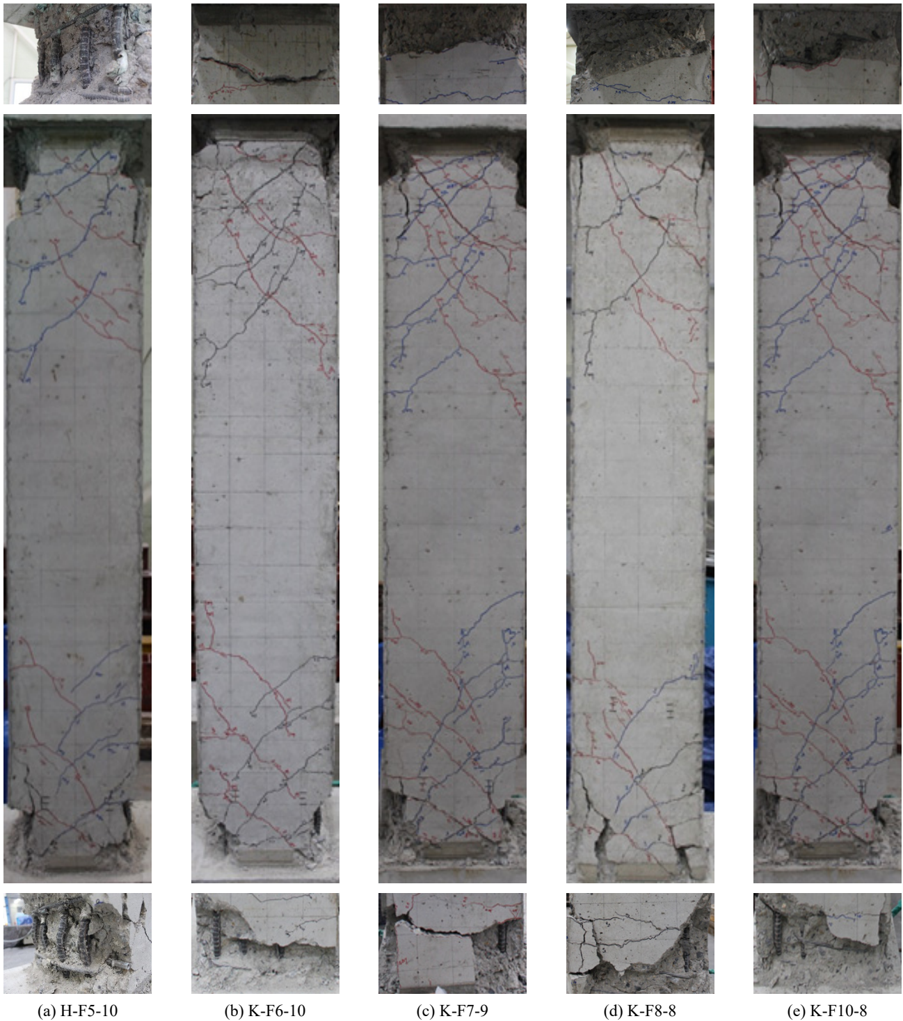
Fig. 6 Crack patterns in specimens at failure
