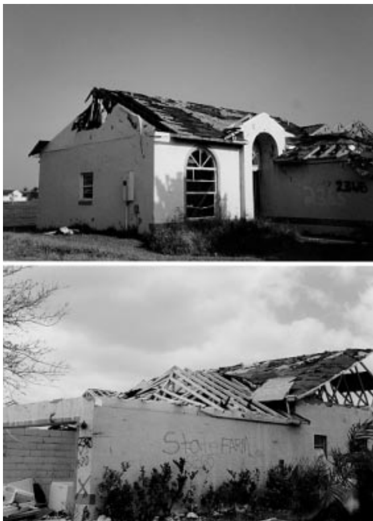
Fig. 10 Views of the south side (top) and north side (bottom) of Case Study 2 showing garage door, roof sheathing and roof structure damages
