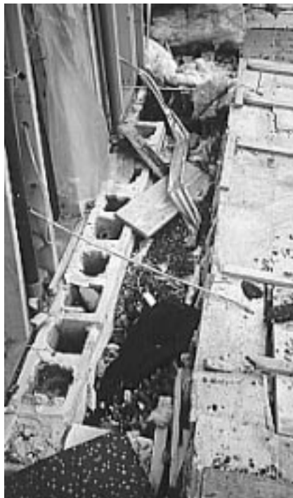
Fig. 4 Insufficient wall to foundation anchorage in the Lakeside Estates
