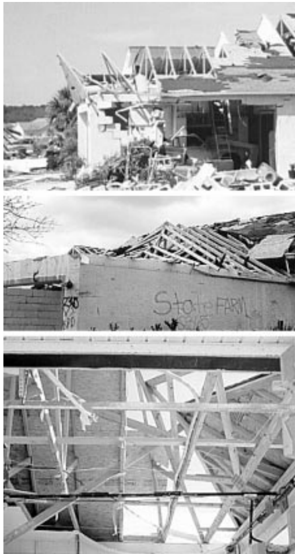
Fig. 3 Deflection of wooden roof trusses due to inadequate lateral bracing (Lakeside Estates)
