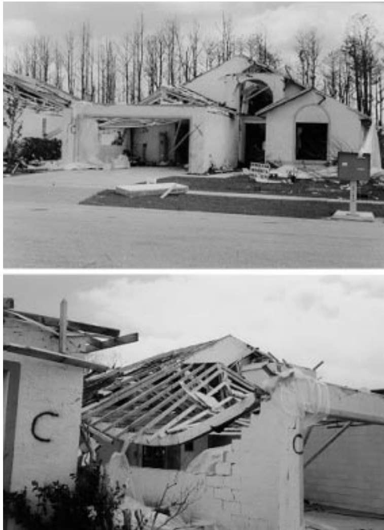
Fig. 11 Front view (top) and side view (bottom) of Case Study 3 showing envelope failures, roof structure failures and masonry wall collapse
