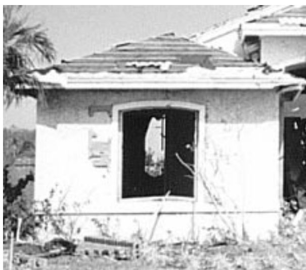
Fig. 1 Window failures in the Lakeside Estates
