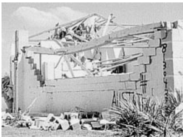
Fig. 6 Bending failure of an unreinforced masonry wall in the Lakeside Estates. Notice that the masonry wall failure caused the tie beam to sag which subsequently led to the collapse of the roof
