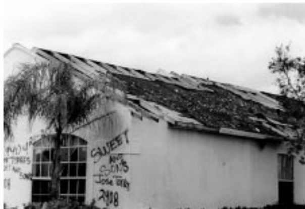
Fig. 9 Rear/side (weat/south) view of Case Study 1 showing window failure and roof sheathing separation at the eaves and along the ridge
