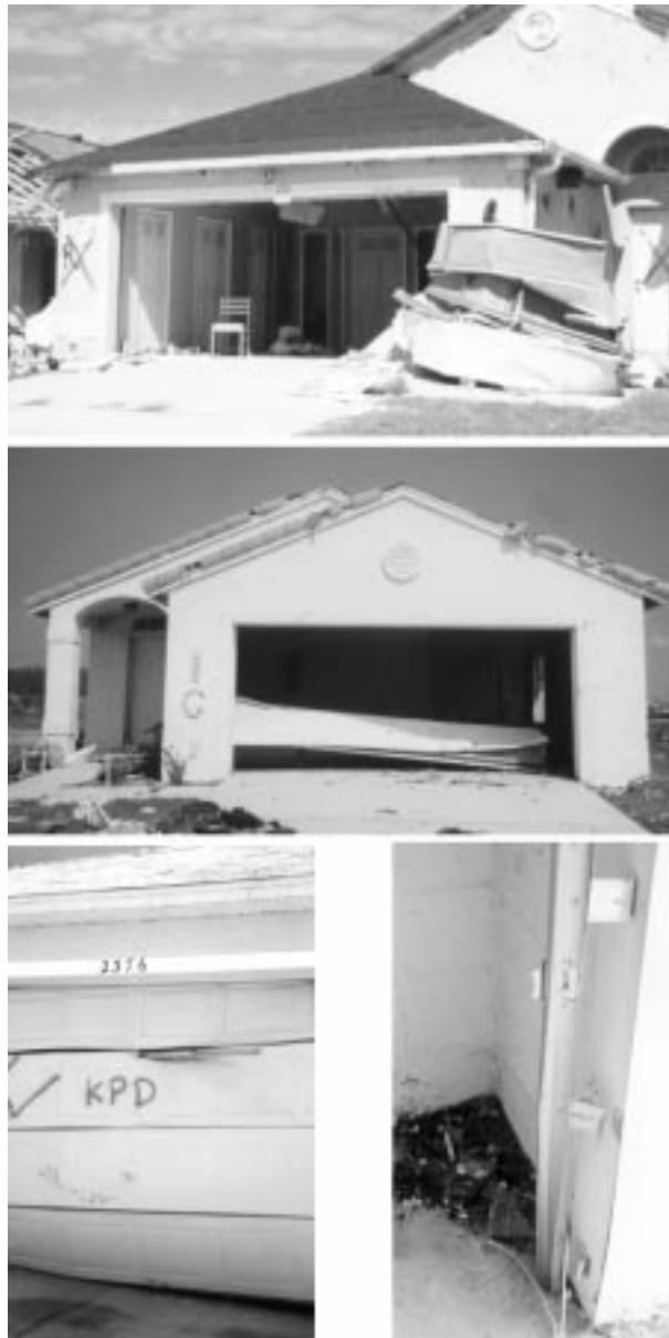
Fig. 2 Garage door failures in the Lakeside Estates
