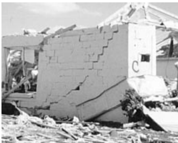
Fig. 5 Shear failure of a masonry wall in the Lakeside Estates
