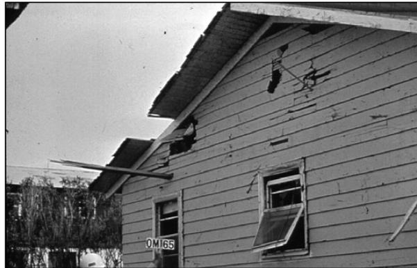
Fig. 1 Debris impact damage (photo by Texas Tech University)
