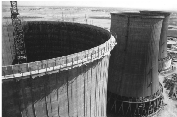
Fig. 1 General view of cooling towers wind ribs
