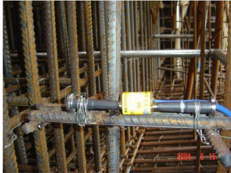
Fig. 3 A vibrating wire strain gauge installed inside the bridge before the concrete casted
