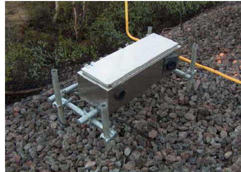
Fig. 15 T/BOGI installation side tracks (Lagnebäck 2007)
