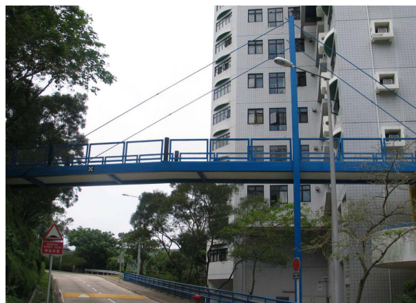
Fig. 9 A single-tower pedestrian bridge
