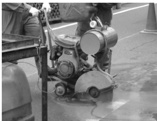
Fig. 2 A road cutter is cutting the road
