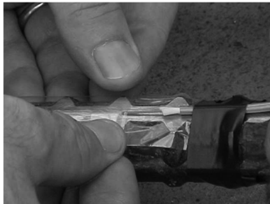
Fig. 4 Installation of sensors on rebars
