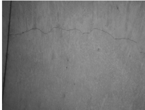
Fig. 9 1st crack on bottom of bridge deck
