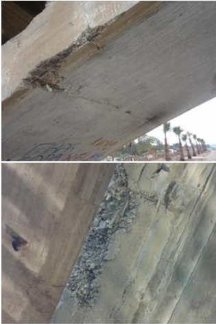
(b) Deteriorations and shell concrete failures
