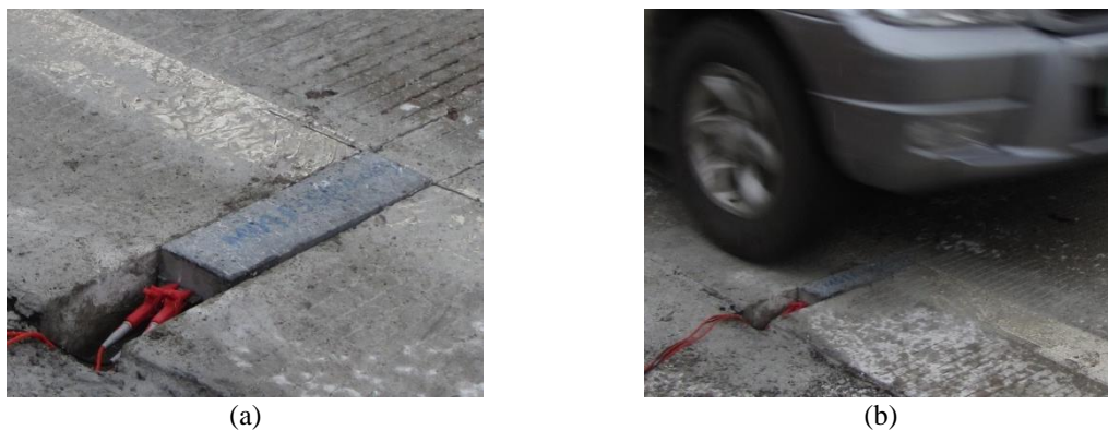
Fig. 9 An installation of the composite sensor in the road pavement (a) and an application of the vehicle wheel load on the sensor (b)
