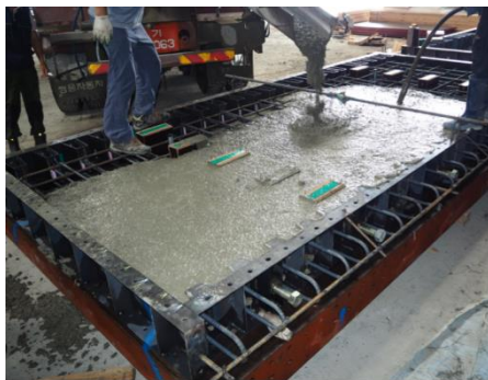
(a) Form fabrication & concrete pouring
