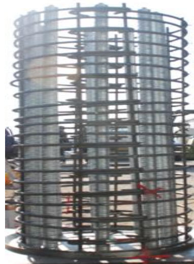
(b) Transverse reinforcement for segment segments
