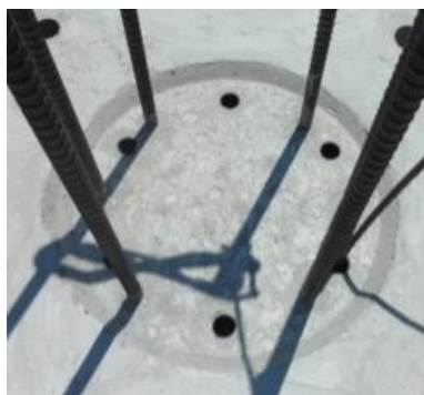
(c) Joint between a segment and footing
