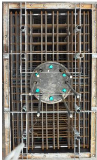
(a) Reinforcement of footing
