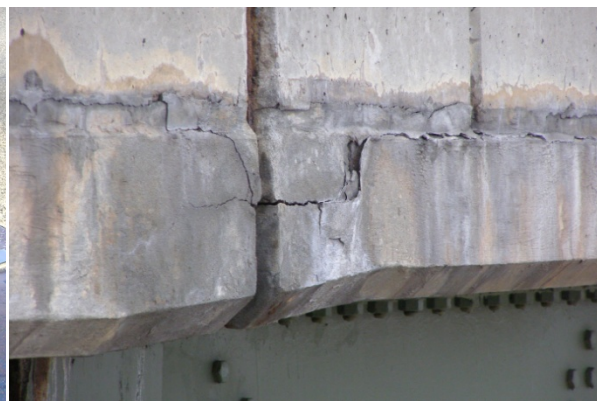
(b) spalling fascia
