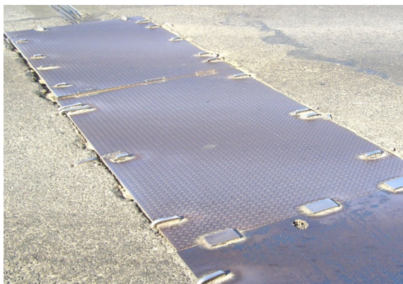
(a) steel plate replacing a failed joint
