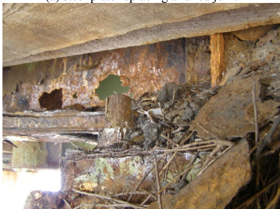
(c) bearings, pedestals under expansion joint
