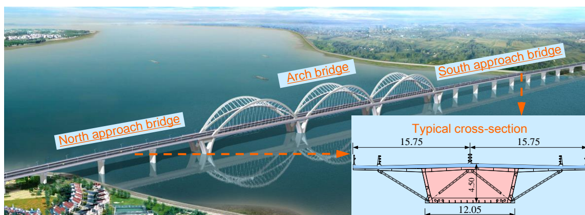
Fig. 1 Jiubao Bridge (unit: m)
