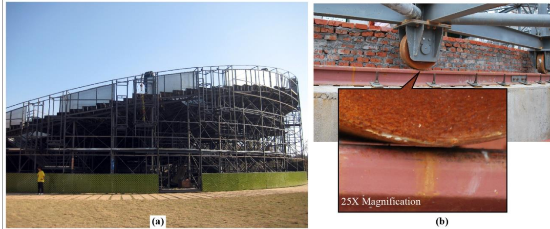
Fig. 14 (a) Photo of revolving auditorium under construction; (b) Photo of wheel-rail detachment
