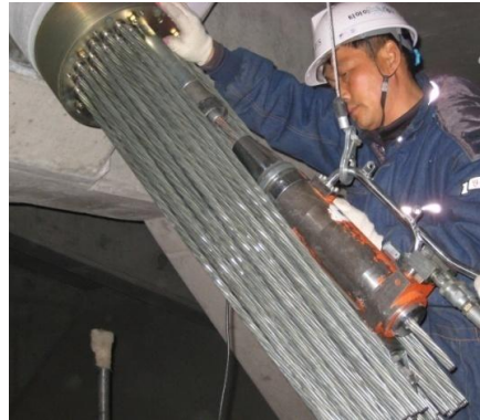
Fig. 7 Cable tensioning work
