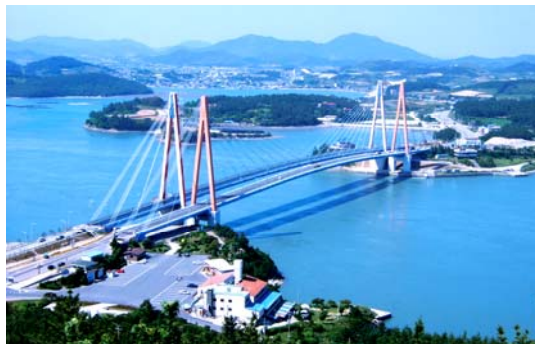
Fig. 12 Jindo Bridges (left is the 2 nd Jindo Bridge with wireless monitoring system)
