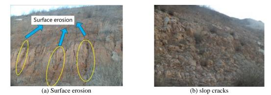
Fig. 3 Surface damage of the cutting slope
