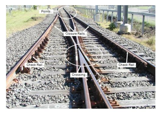
Fig. 1 Typical turnout structure and geometry
