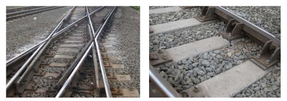
(a) pulverised ballast and broken concrete sleeper due to poor energy dissipation of material
