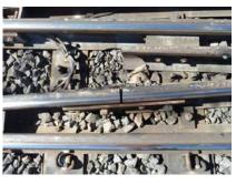
(f) a joint gap at a mechanical joint
