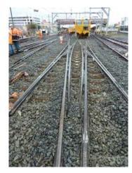
Fig. 9 Double slips installation and resurfacing
