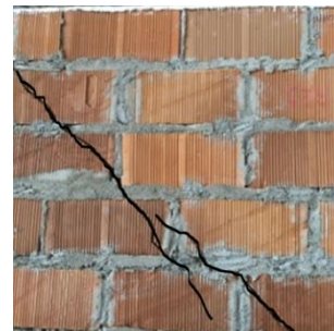
Fig. 4 Damages of the cement mortar walls
