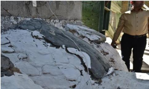
(a) FRP cement sand mortar separated from the rib cover
