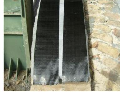
(b) Installing CFRP
