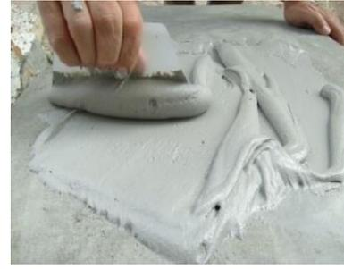
(a) Application of thin layer of primer to the surface
