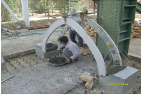
(a) Installation of the plaster stencil as a template
