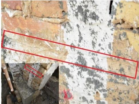
(b) Cracks at the closest point to the spring
