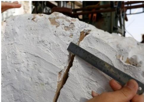
(c) Increase the width of the cracks in the right vault to 2 cm
