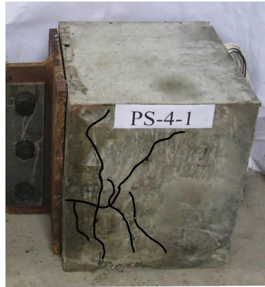
(a) Crack of concrete slab
